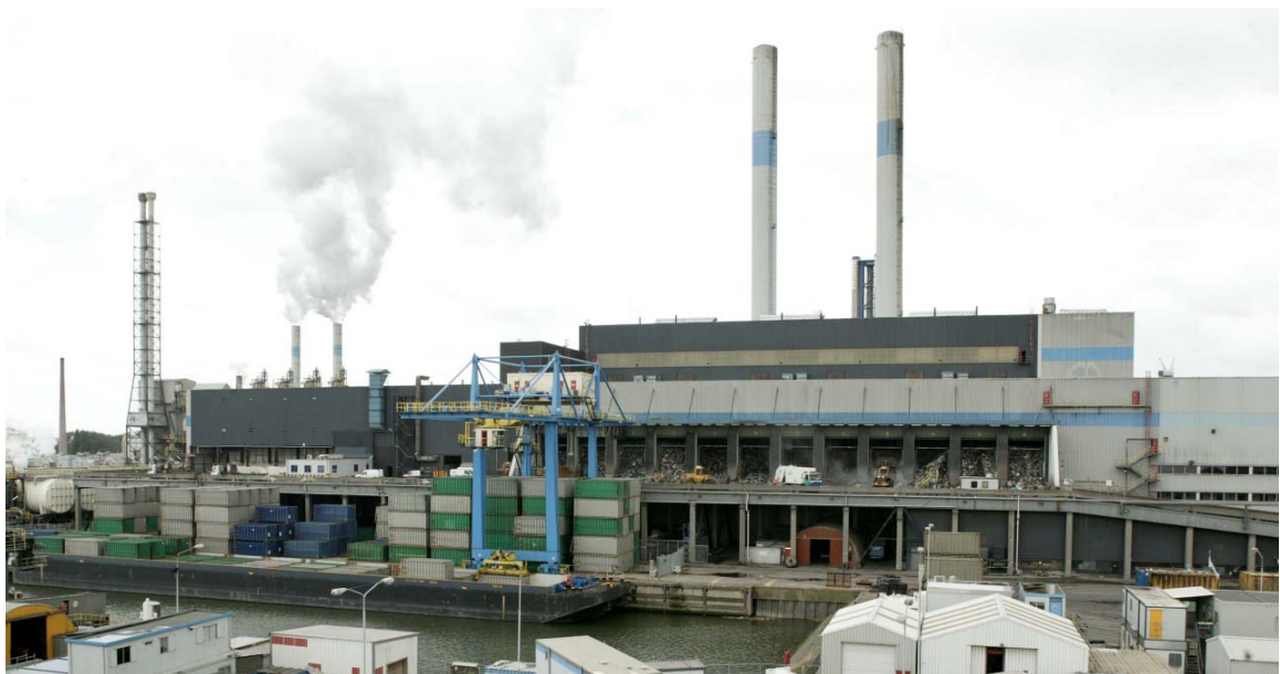
Processing plant at AVR Rozenburg
